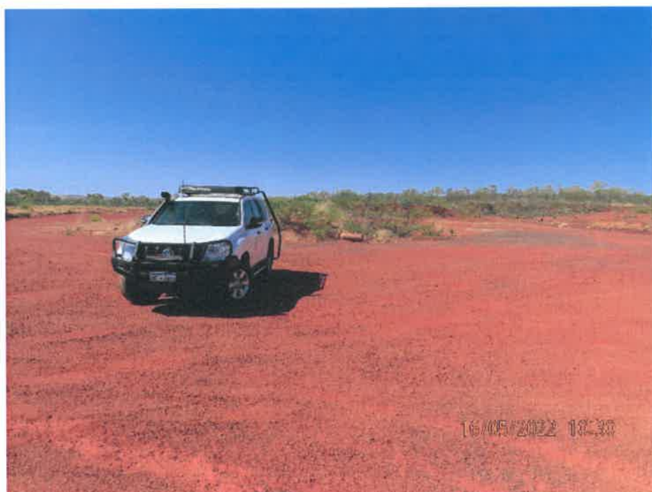
Figure 7 View of the earth bank-GNH
