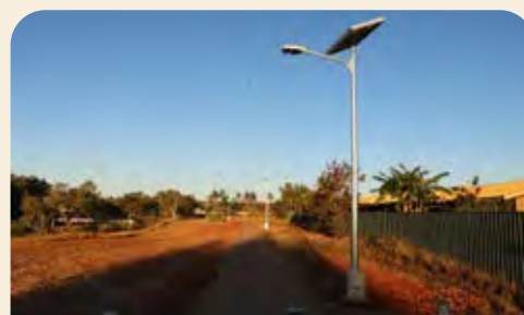
Upgrade Footpaths and Lighting
