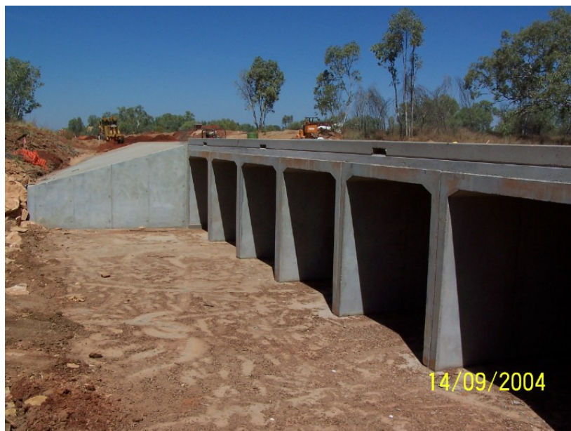
Construction of Culverts for the Sturt Creek Bridge
